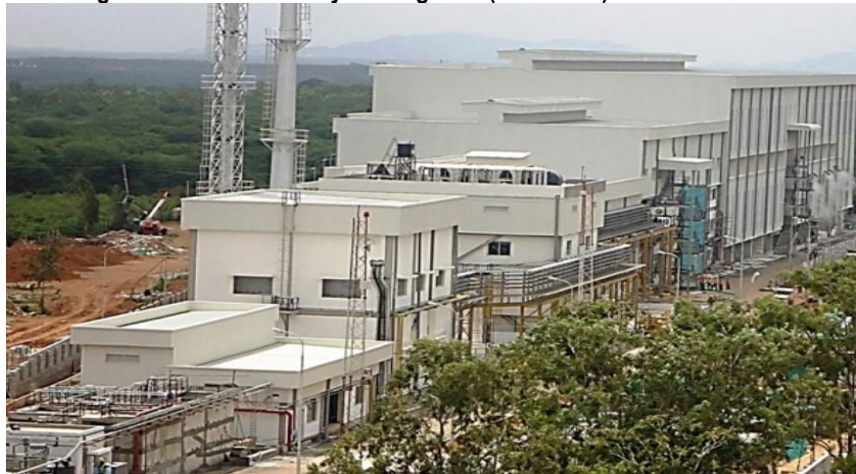
Fig 29 – JSSL undertook designing, metal decking, roofing/cladding and Tekla modelling for ITC noodle factory in Bengaluru (Karnataka)
