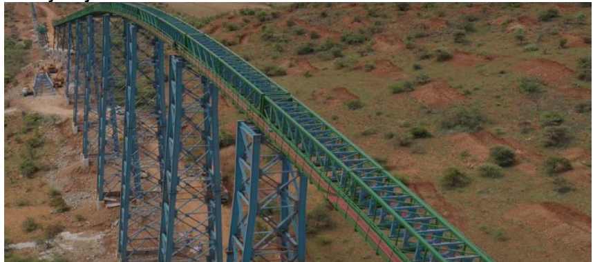
Fig 19 – ~3,500 tonnes of ore can be transported per hour, world's largest pipe conveyor system
